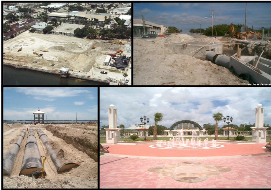
Stormwater reuse retrofit project in Cocoa, FL serving a 12-acre downtown drainage basin. Photos courtesy of Eric Livingston.
